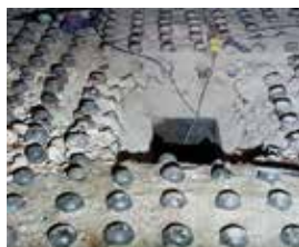
Fig.7. The rectangular bottom ash discharging outlet and the arrangement of the wind caps.
