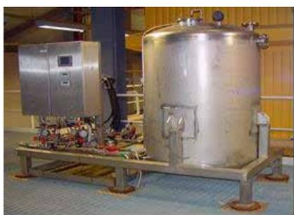
Fig.3a. Overview dosage system and intermediate storage tank
