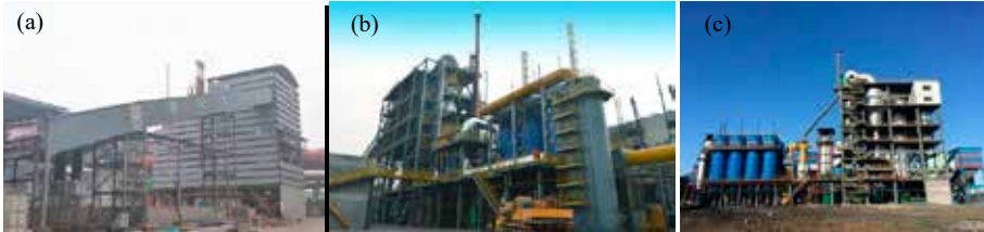
Fig.2 Pictures of industrial CFB gasifier: (a) 25000 Nm 3 /h hot flue gas production (Jiangsu Huiran); (b) 40000 Nm 3 /h cold flue gas production (Xinfa huayu-stage I); (c) 60000 Nm 3 /h cold flue gas production (Jiujiang jiaohua)
